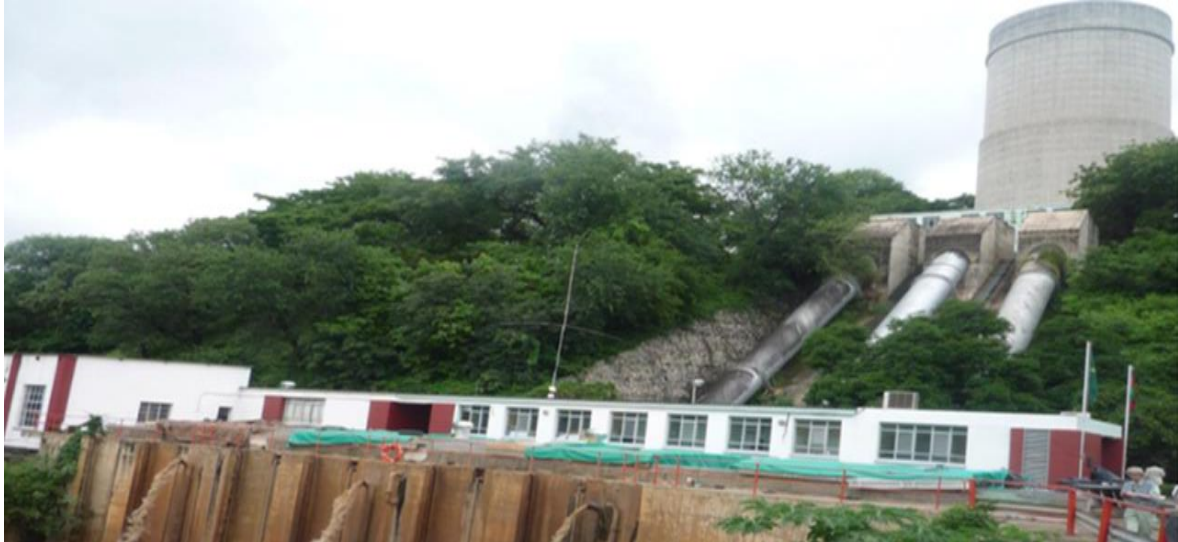
Figure 1: Nkula Hydro Power Plant
