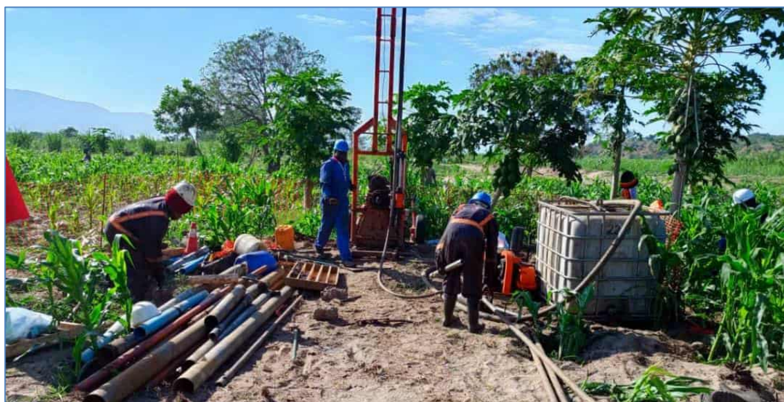
Figure 13: View of Geotechnical Investigations during the Basic Design
