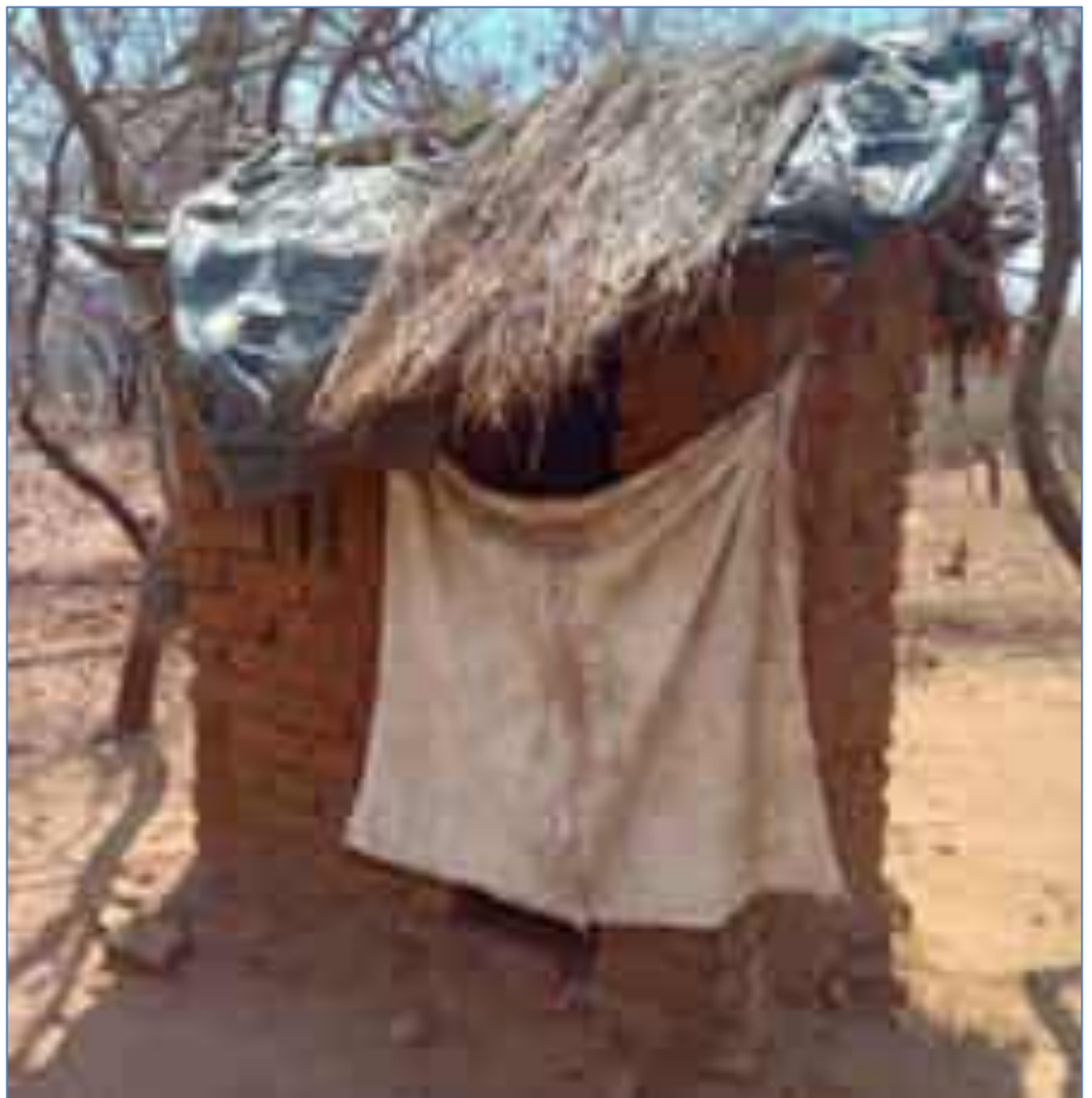
Figure 102: Typical Latrine (Feremu, Neno District)
