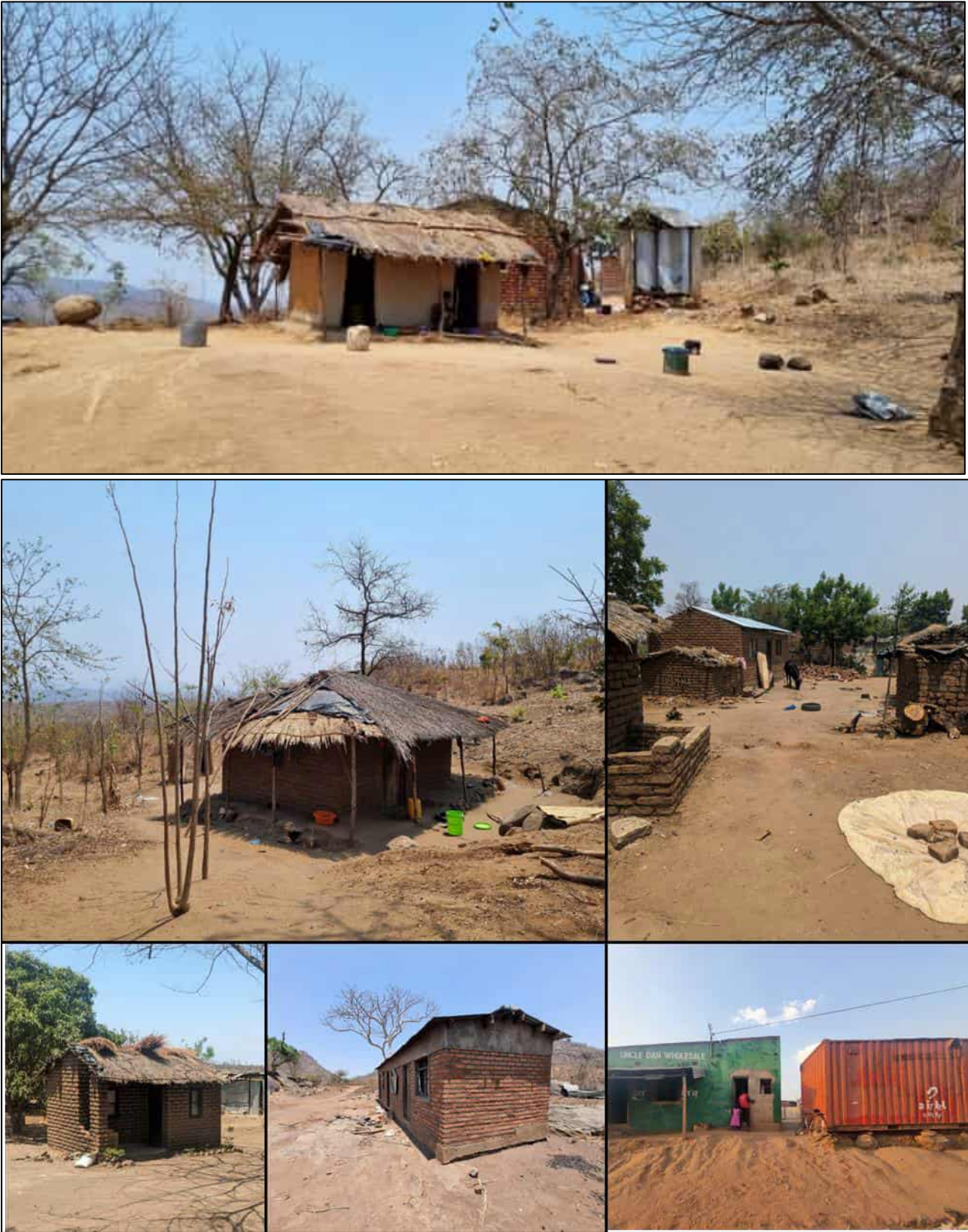
Figure 87: Typical Housing Structures within the Study Area
