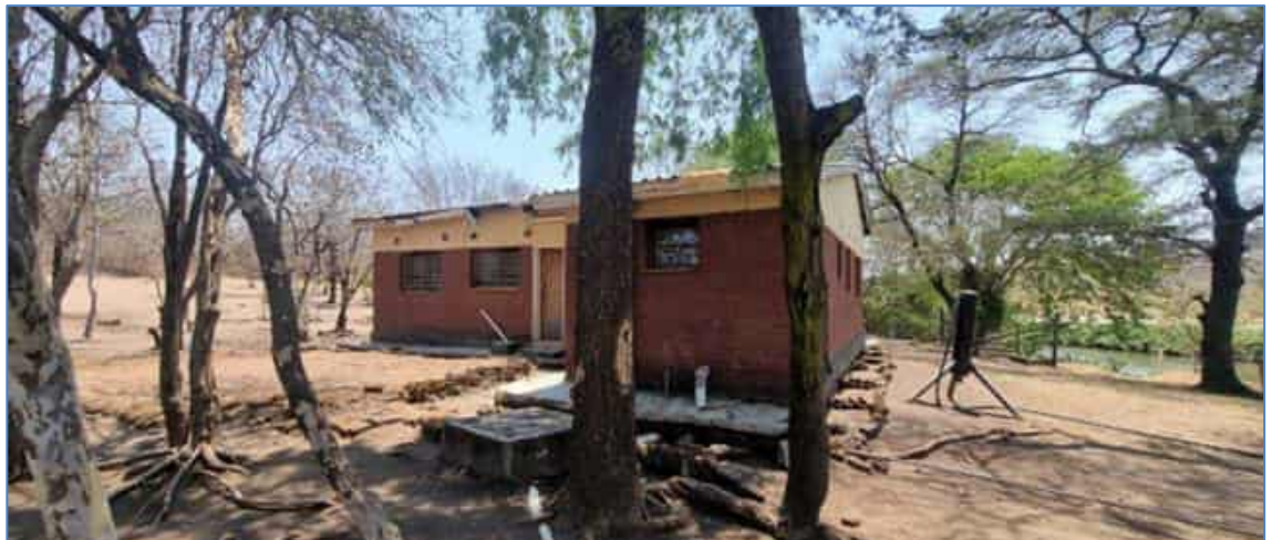
Figure 83: Ranch workers accommodation on Zagaf ranch
