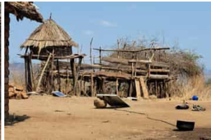
Figure 67: Poultry Housing ( Khola ) on the Left And Goat, Ducks and Sheep Housing, Near Houses in Chinkwynia Village (Blantyre District).
